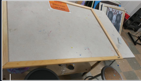
- Creating the wooden frame.
